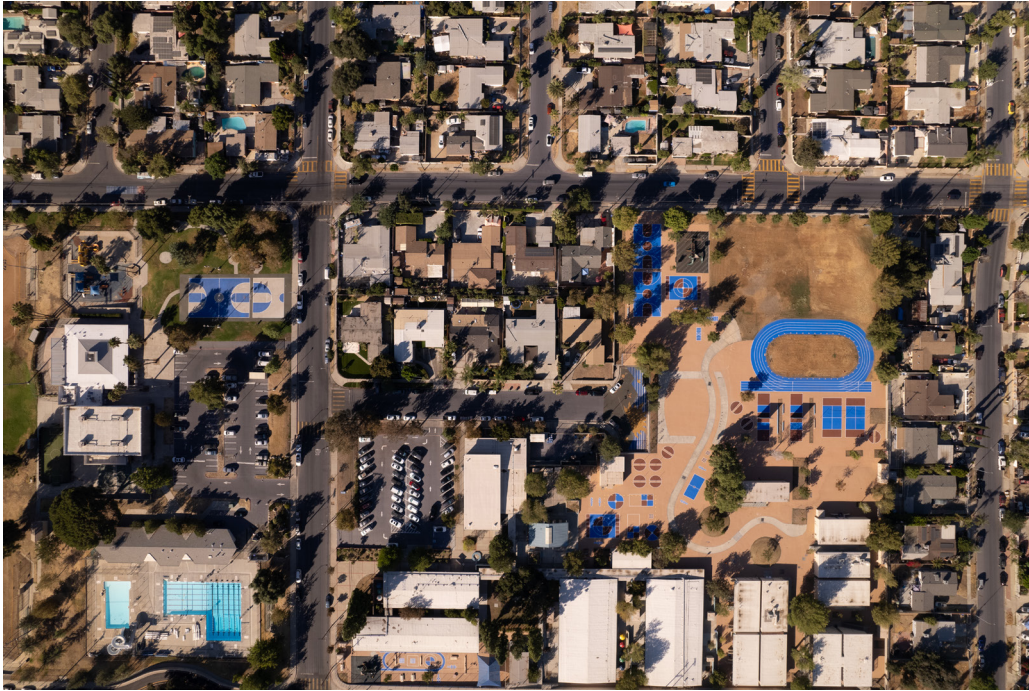
Aerial photo showing the different types of surfaces after coating
