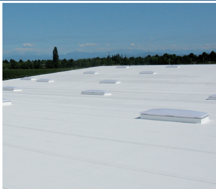
White roof membrane
