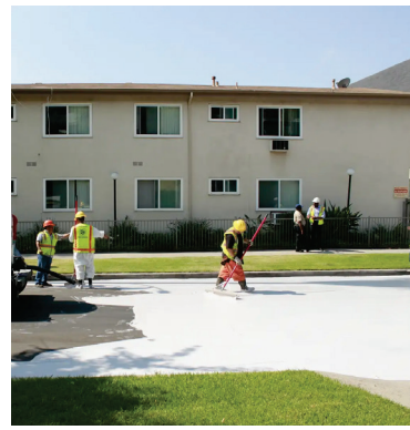
White pavement coating
